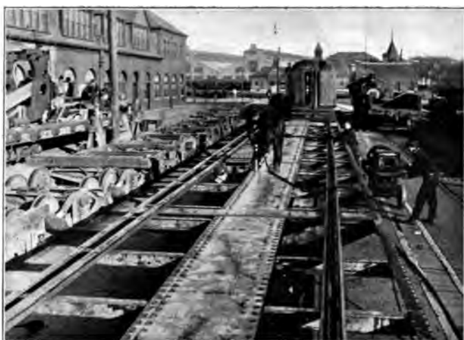
Riveting the underframe
